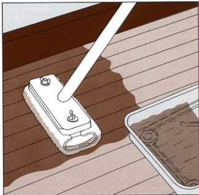
Fig. 8. A long-handled lamb's wool applicator is excellent for applying penetrating seal finishes or pigmented wiping stains. Spread generously in the direction of the grain; wipe up excess.
