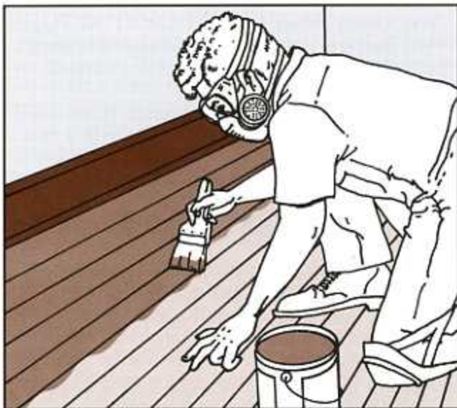
Fig. 9. When using a brush to apply a surface finish, work in the direction of the boards in a path narrow enough to keep a wet edge. Lap strokes back into area just covered.
